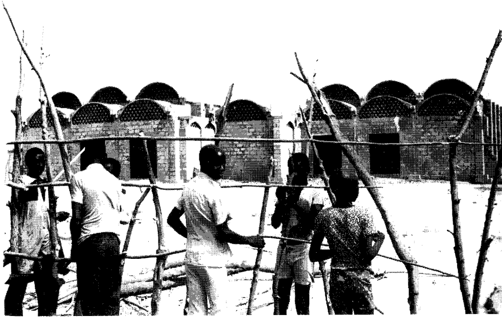
ABOVE: Students building a fence to surround the new, World Bank-funded EMP center at Nguékokh, Senegal. BELOW: Posing in the garden of the EMP program in Bargny, Senegal.
