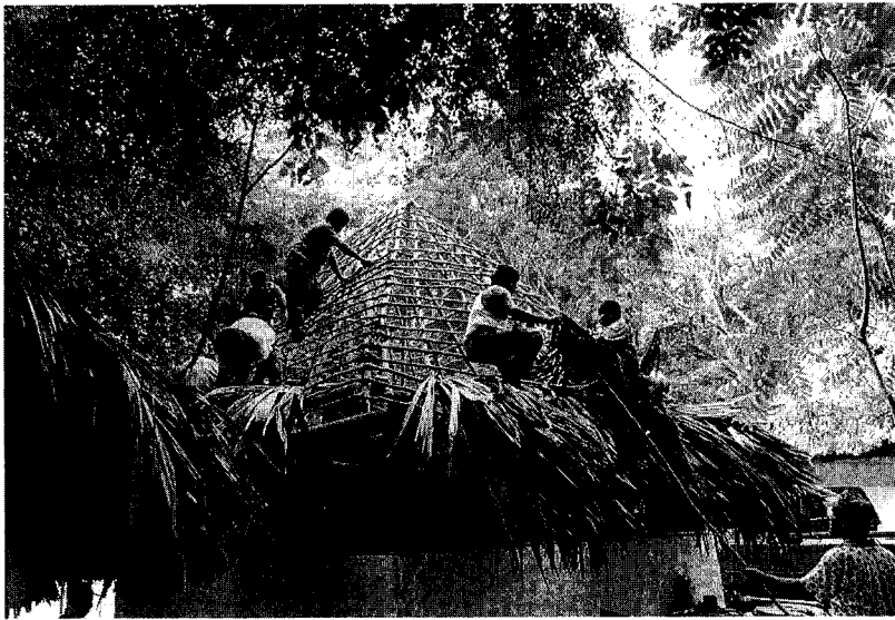
CONAP Park guards constructing a roof with guano palms
