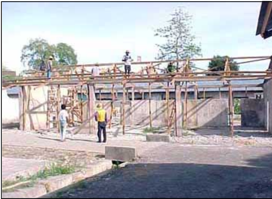
Rebuilding the market in Suai.
