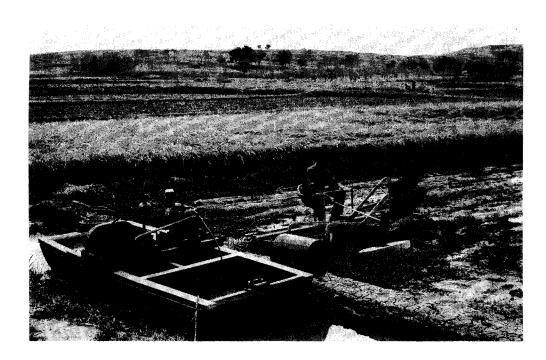
The cable towed plough. Demonstrated outside the Agricultural Mechanization Research Institute, Nanking. The winch on this boat is powered by an electric engine.
