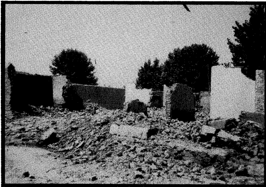
Only rubble remains where houses stood three months ago.
