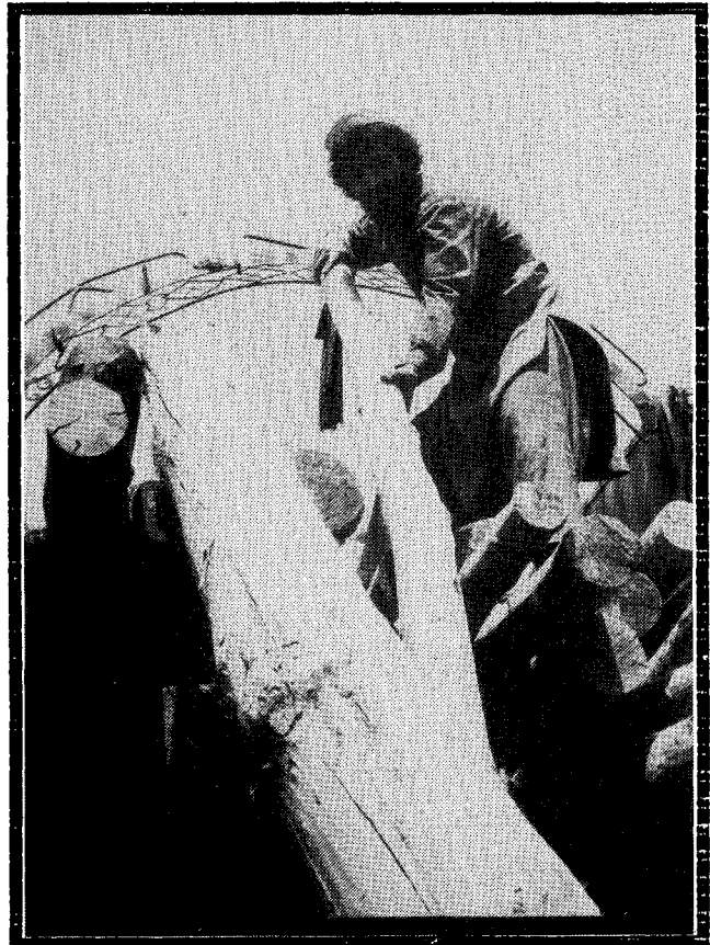
An Afghan loads wooden roofbeams on to a truck in preparation for the reconstruction of his home in Afghanistan.
