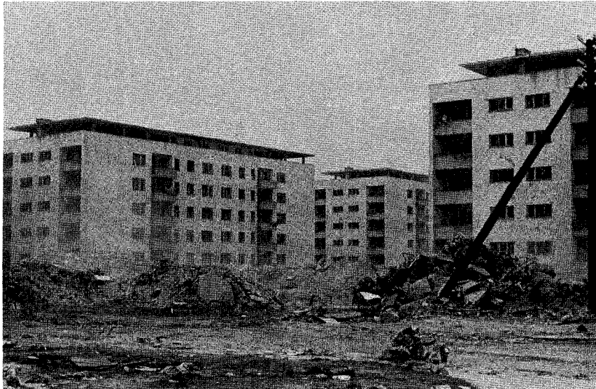
KARPOŠ: In this modern subdivision, one apartment house collapsed completely, with 195 dead. Others, while they looked complete except for windows, were so structurally shattered that they must be pulled down. On abandoned balconies potted plants slowly shriveled and died in the hot sun from lack of attention, mute symbol of the death of the city.
