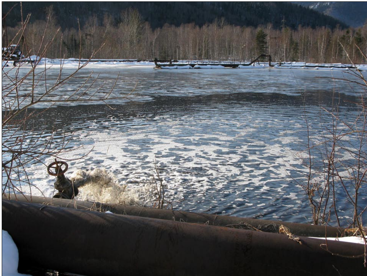
As I roamed around the plant's storage tanks last November, I saw rusty pipes and leaks everywhere.
