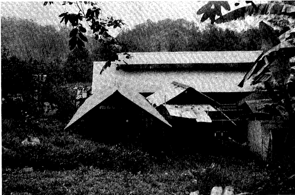
Cooking facilities beside the students' dining room (at right), Abepura.
