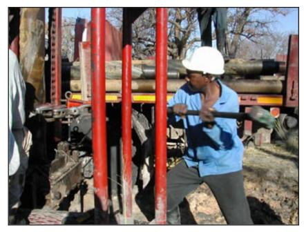
**If stuck, force it**: *John Sr. swings a sledge to unscrew the drill bit. It was later loosened by a blowtorch heating the joint.*
