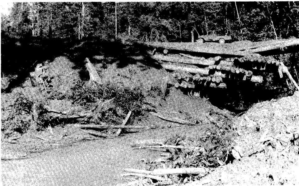
Log and earth bridge on main logging road (pick-up wreck on left side)
