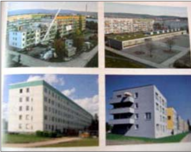
The top two photos show a plattenbau that was dismantled and rebuilt as a row of duplexes. The bottom two photos show a five-story, 650-foot-long plattenbau rebuilt into a row of eight “city villas”.
