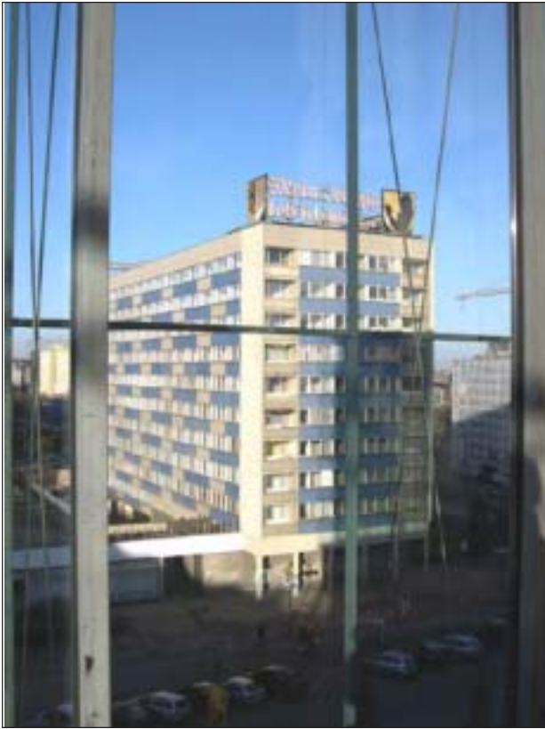
A view of one of the crumbling East German high rises across the street from the brand new Museum of Visual Arts in Leipzig.
