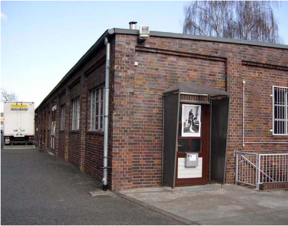
This obscure brick structure on a lot filled with industrial buildings is the unlikely home of Peres Project's Berlin outpost.
