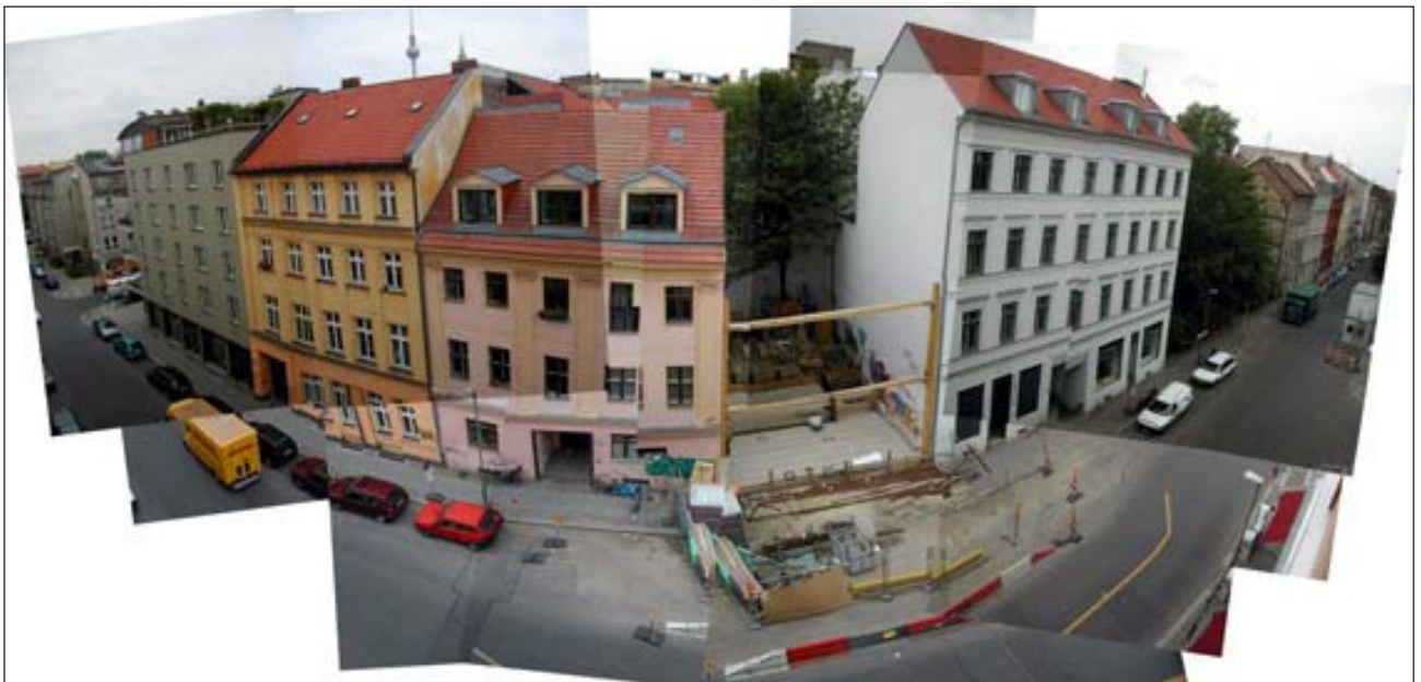
View of the lot during construction. Photo: Jörg Ebers
