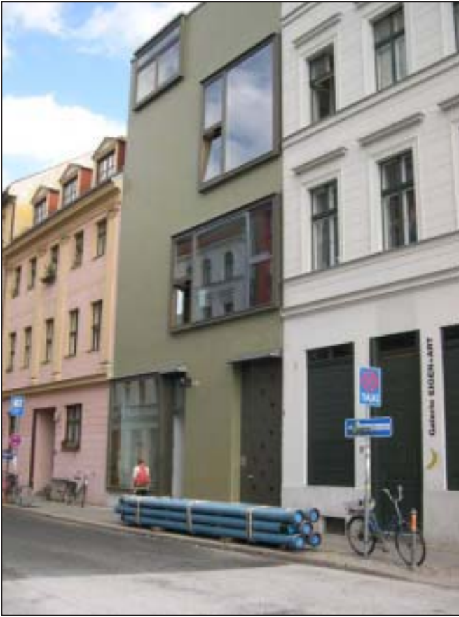
View of Ebers's building, located in between a renovated early-20 th -century house and the renowned gallery EIGEN + Art (to the right).
