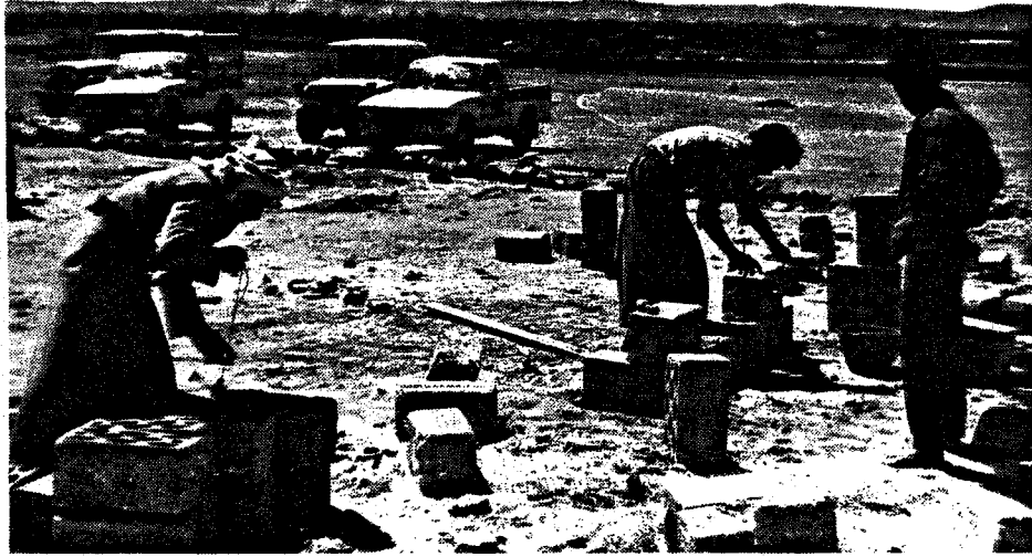
Yemeni masons learning new earthquake-resistant building techniques at Oxfam's Dhamar training center. The man at right is a Yemeni Oxfam supervisor.
