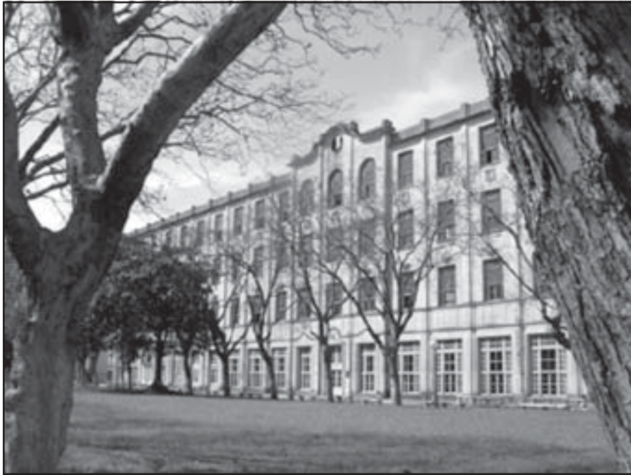
The front of the Immigrants' Hotel, located right next to the dock at the port of Buenos Aires
