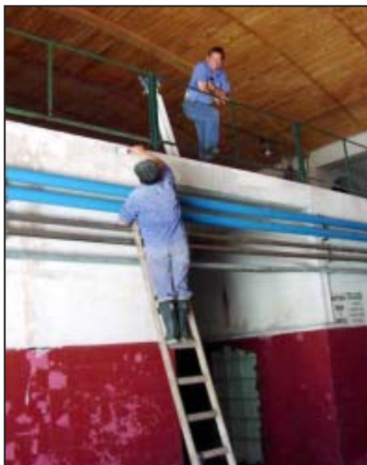
Painting one of the massive holding tanks in the Michel Torino winery.
