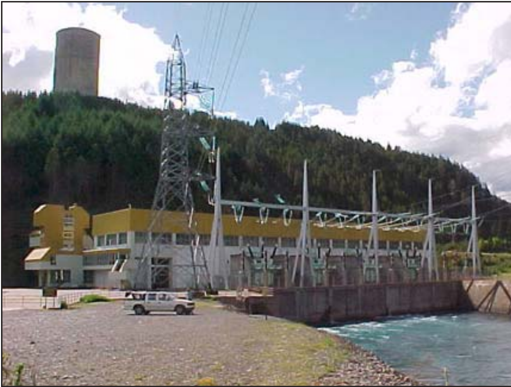
The Argentina-based Hidroeléctrica Futaleufú Inc. generator house, where the Futaleufú River now begins its free-flowing state toward Chile and into the Pacific Ocean-
