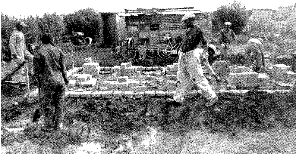
Bricklayers start construction on a standard two-room house.
