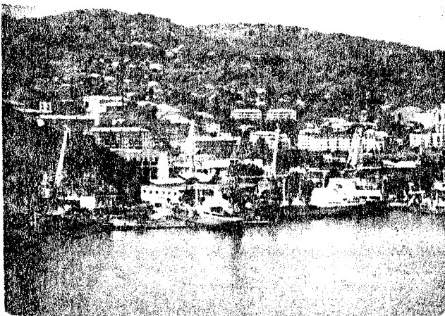
One of the residential districts adjacent to the port.
