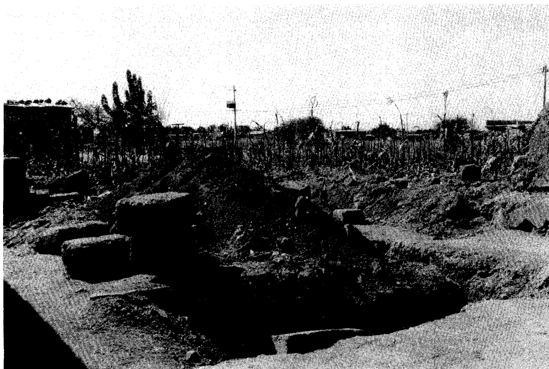
The remains of houses in Ga-Pila that were destroyed by "flyrocks" and the earth's vibrations caused by PPL blasting
