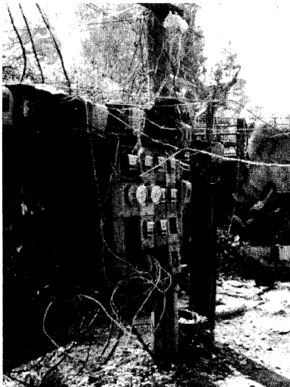
Illegal wires hung from electricity meters to "hijack" energy from Central Power and Light
