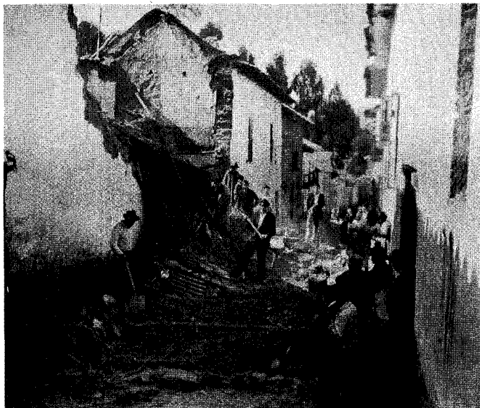
..... Street scene after 1950 'quake. Note buried truck in center .....
