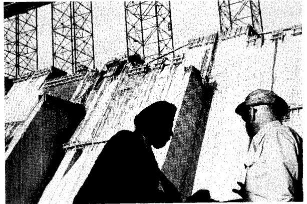
BHAKRA DAM: Indo-American confab
