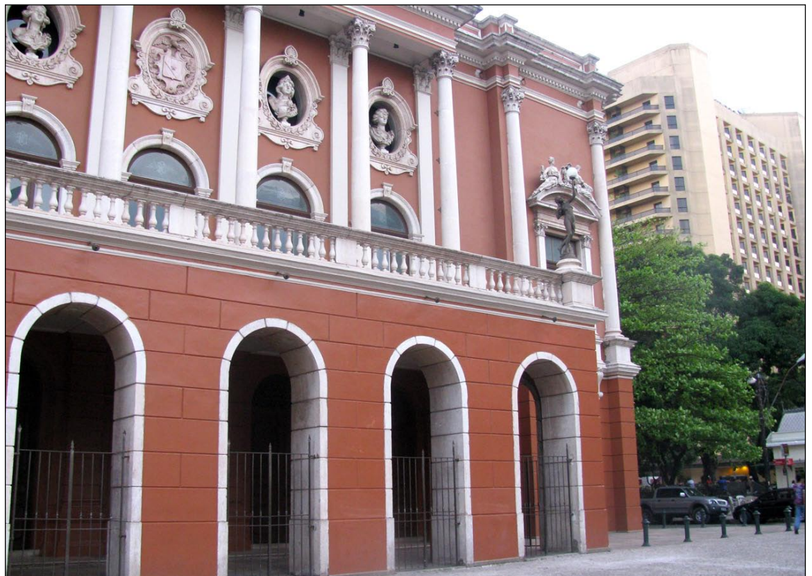
Belém’s “First World” architecture: the neoclassical Teatro da Paz and 1970s concrete monstrosity Hilton Hotel surrounded by the city’s timeless mango trees.
