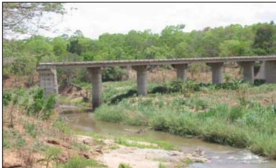
A bridge in Zambézia Province, destroyed by Renamo rebels. Reminders of the long civil war are everywhere in Mozambique.
