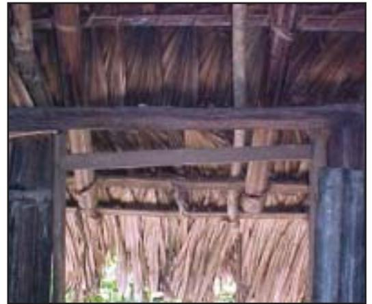
*(Top, left) The ceiling of Silverio's house is a masterpiece of geometry. (Top, right) In this photo of the eaves around Silverio's doorway, one can see wood from seven types of tree. (Right) The main room of Silverio's house. With walls of bebak and shingles of tali fronds, his home is a monument to the sago palm.*
