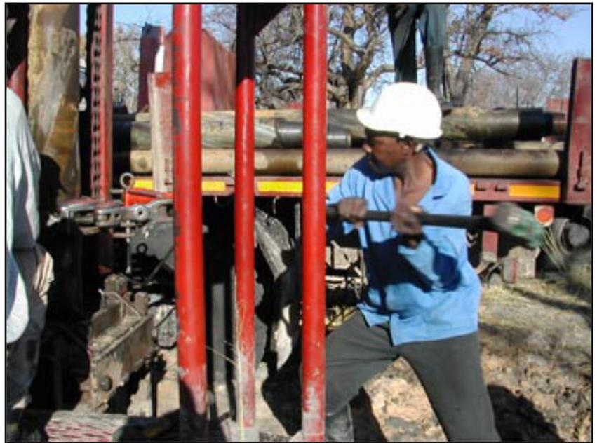
**If stuck, force it:** John Sr. swings a sledge to unscrew the drill bit. It was later loosened by a blowtorch heating the joint.
