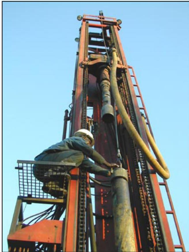
**Avast Up Thar Matey:** A Prinsloo drilling-crew member leans out of the crow's nest, uncouples the baling clamp and prepares to screw in a drill-pipe segment.
