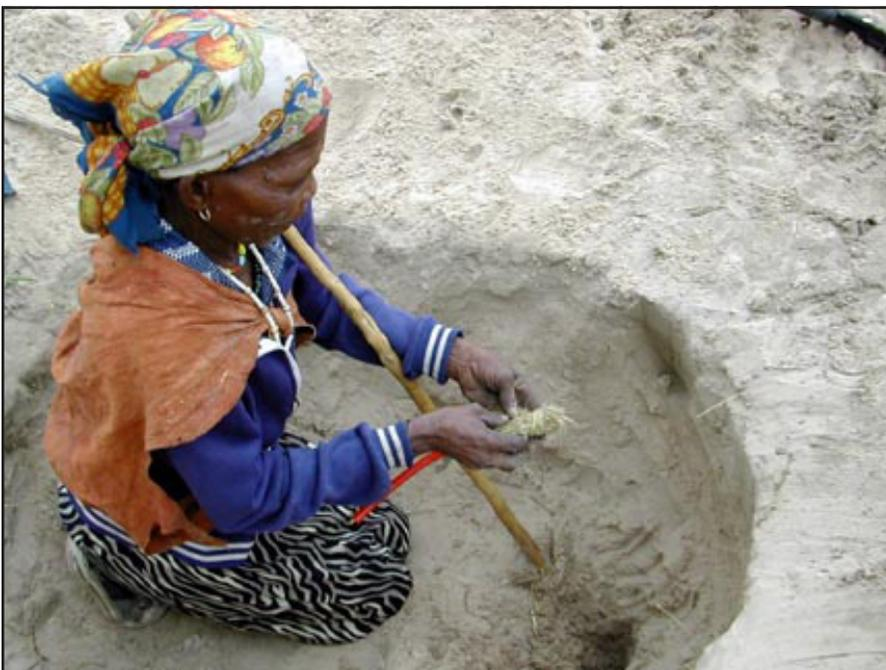
*New Rubber, Old Technique: Thaleta fastens the traditional grass-filter plug to the modern red tube*
